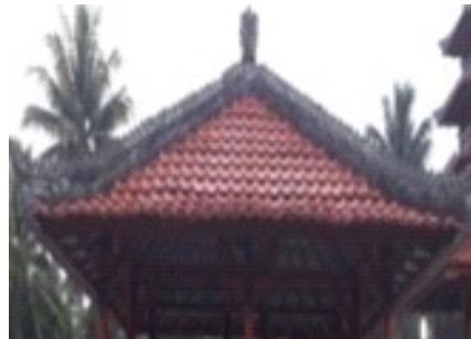
Figure 3. Example of Pelinggih Roof
