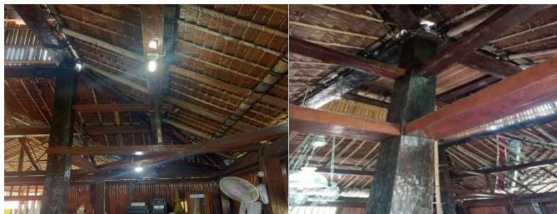
Figure 4. Wooden Anchoring and Connecting the Roof of the Wapauwe Kaitetu mosque
