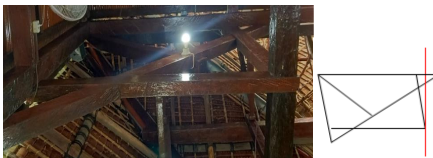
Figure 10. Triangles on the first four corners of the roof
