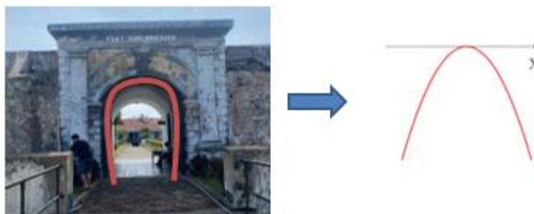
Figure 4. Fort Marlborough gate
